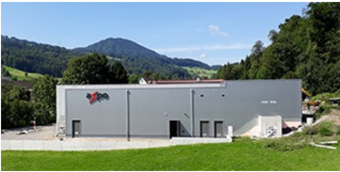
Figure 12: Axpo's Etzel substation in the Swiss Alps
