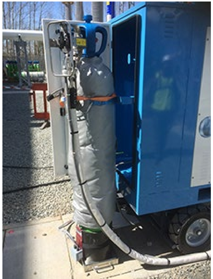
Figure 6: g 3 cylinder with warming system
