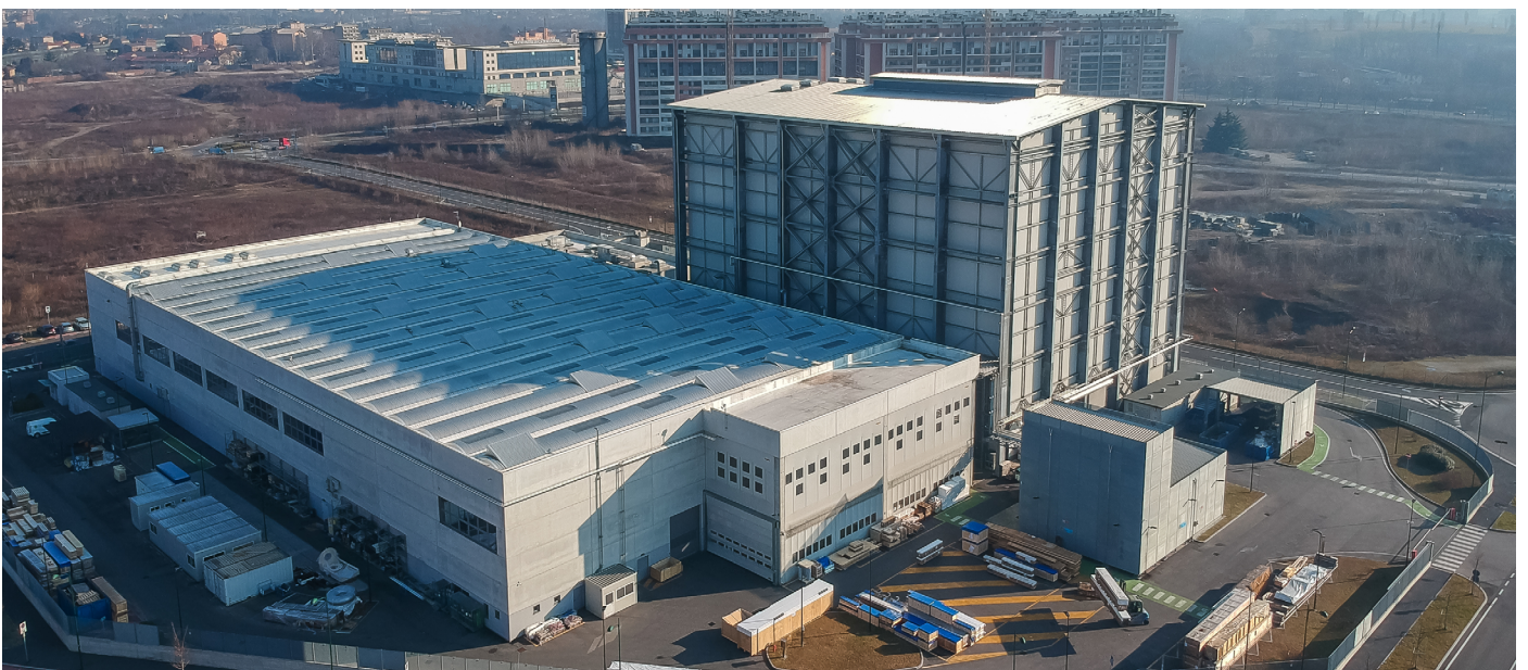
Manufacturing Site: GE Grid Solutions, Sesto San Giovanni, Milan, Italy
