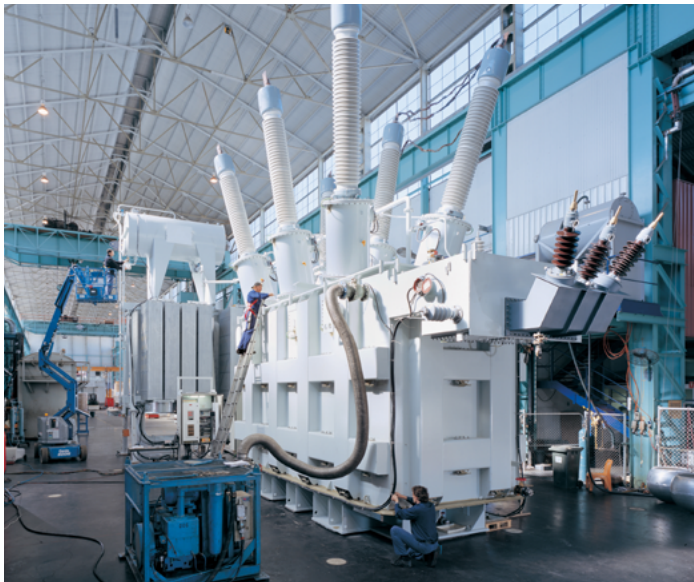
Manufacturing of a 1125 MVA 330/275/33 kV autotransformer for Middle Ridge s/s (Australia)
