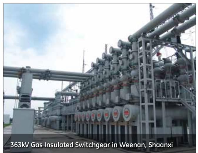
363kV Gas Insulated Switchgear
