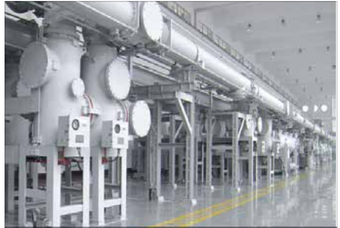
550kV Gas Insulated Switchgear
