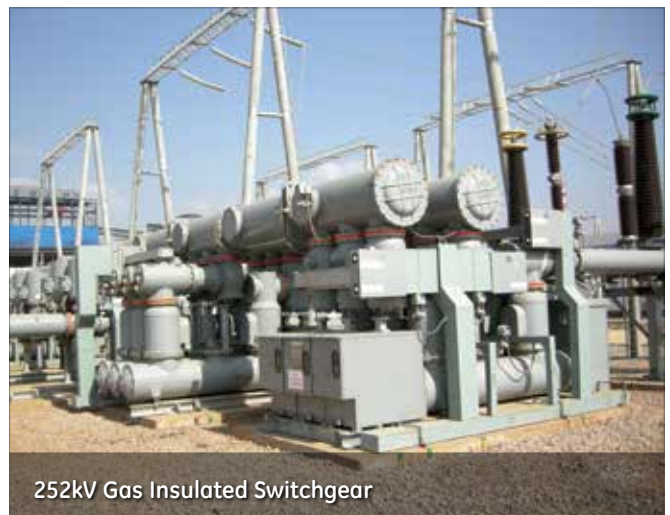
252kV Gas Insulated Switchgear
