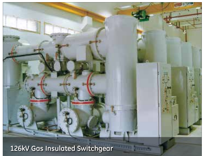
126kV Gas Insulated Switchgear
