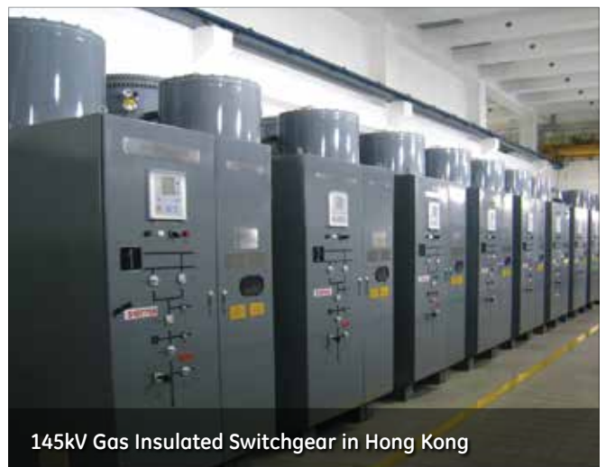
126kV Gas Insulated Switchgear
