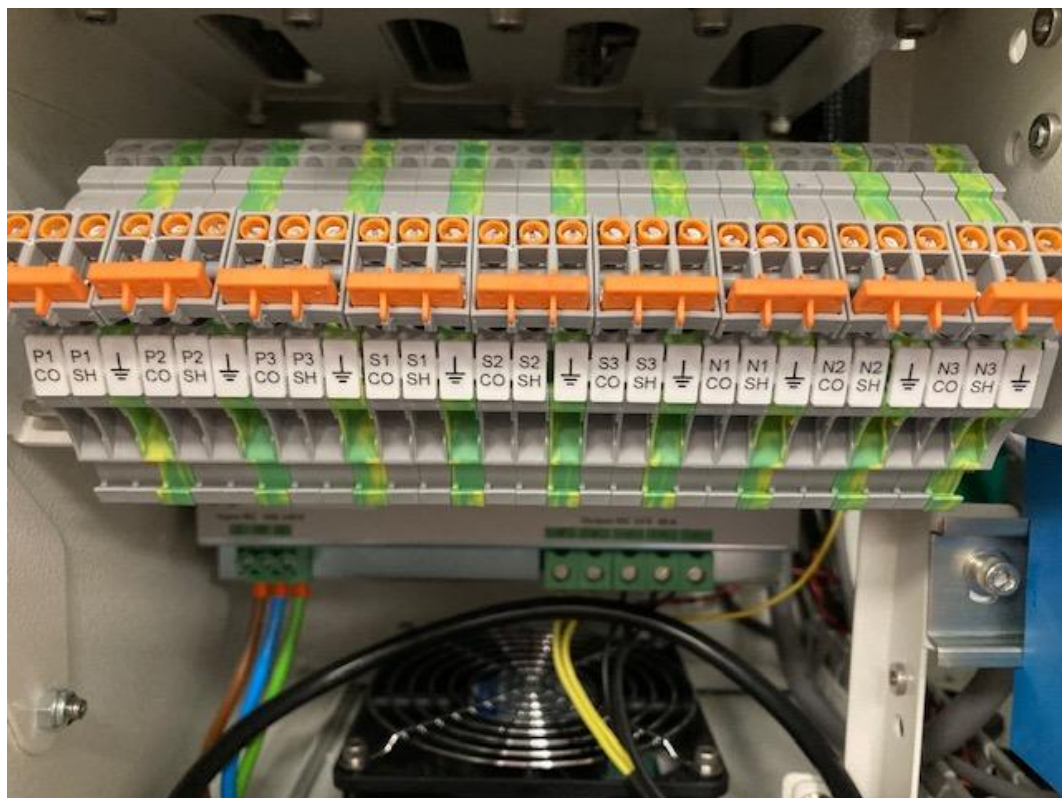
Figure 9-23: Bushing adaptor connections
